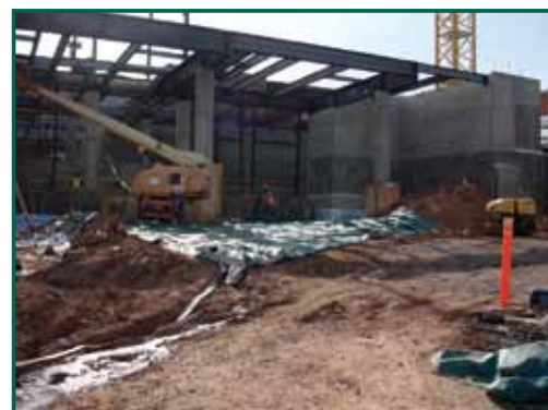
The underground parking structure is now easily identified.
