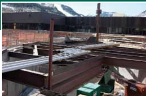
Structural steel that will form the expansion of the patient care unit was placed in the fall of 2011.
